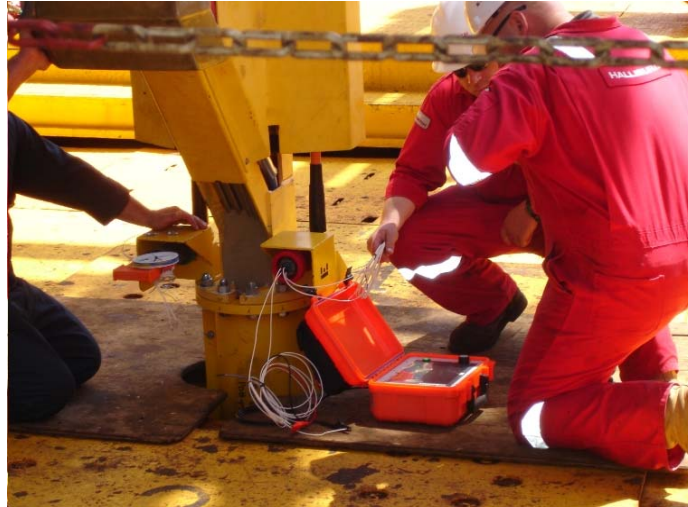
Figure 9: Pre-second end UTA overboarding testing
