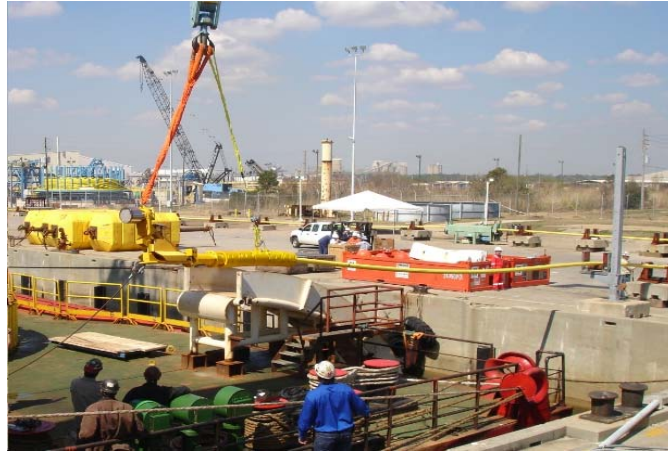
Figure 6: UTA transfer shore to vessel
